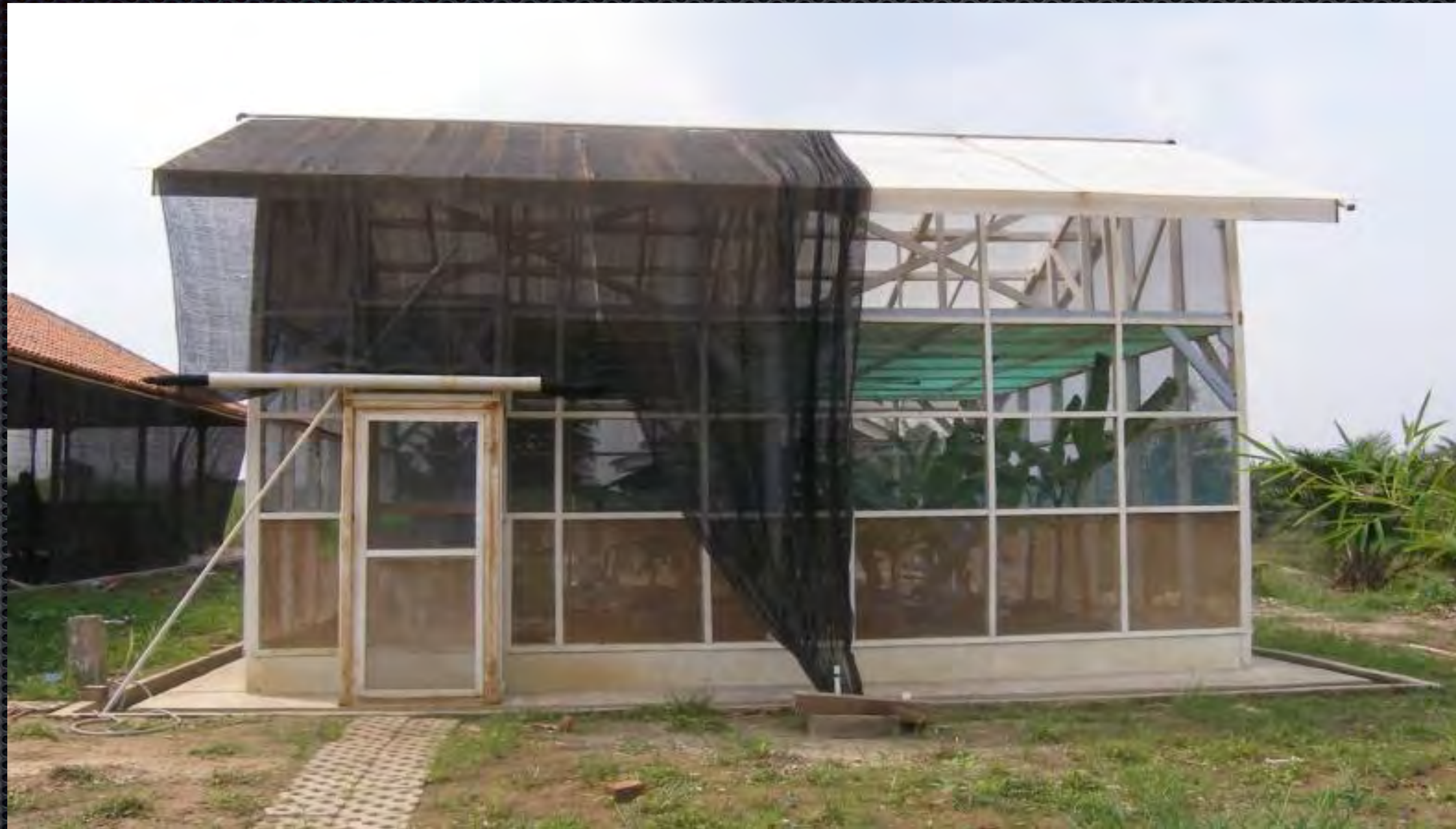
REARING HOUSE, Lampung
